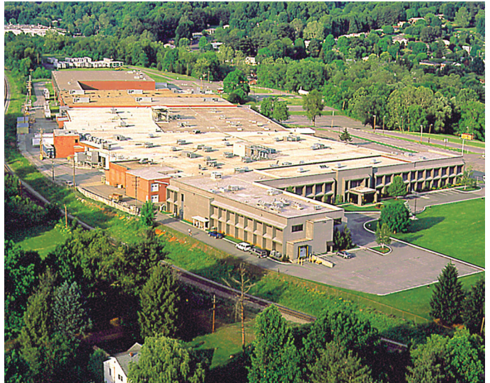
AERUS MANUFACTURING PLANT | BRISTOL, VA
